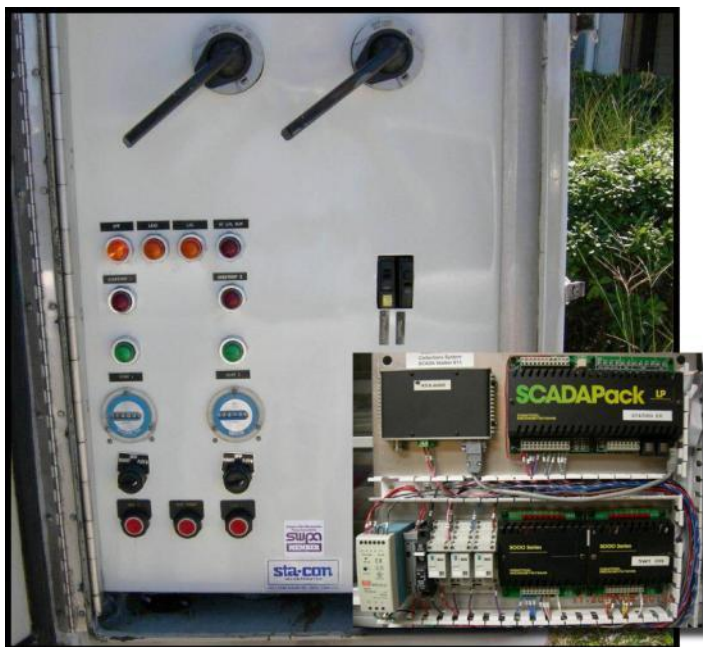
Site Panels designed and built by David Kanoy
