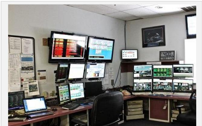
A common HMI streamlines the operator screens of disparate legacy turbine and auxiliary control systems. All changes are immediately distributed throughout all the computers
